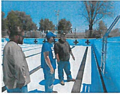
Water Superintendent Nathan Schultze learns about the care and maintenance of the new pool liner from installers from Ren-O-Sys Corp.
